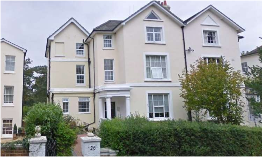
Figure 6. No. 26 Donnington Square showing (original) hipped roof over set-back entrance/stair wing (Image: Google)
